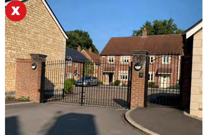
Figure 94: An example from elsewhere in the UK of a formal, high brick and iron gate design which does not represent the rural character of Hartley and therefore similar designs should be avoided.
