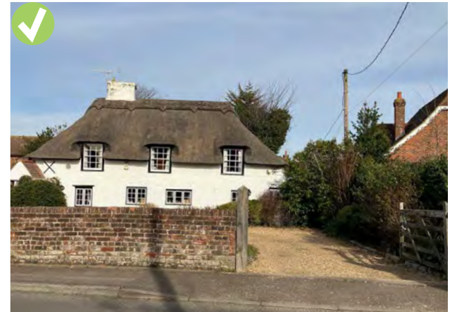
Figure 95: Low brick wall with a wooden gate, an example of a hard boundary treatment which still fits within the rural context.
