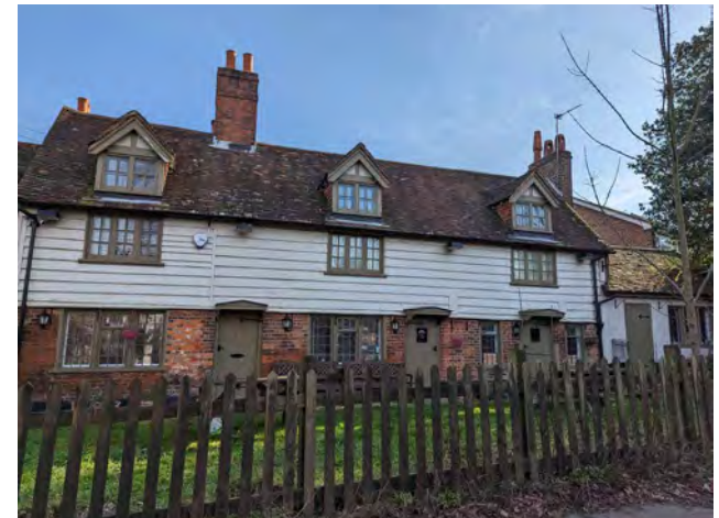
Figure 98: Example of the local architecture of Hartley: weatherboarding, red brick, clay tiles and smalls dormer windows at The Black Lion.
