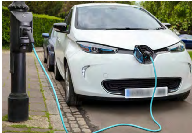
Figure 51: Example of an on-street electric vehicle charging point, elsewhere in the UK.
