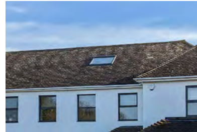
Figure 26: Hipped roof with clay tiles and a skylight.
