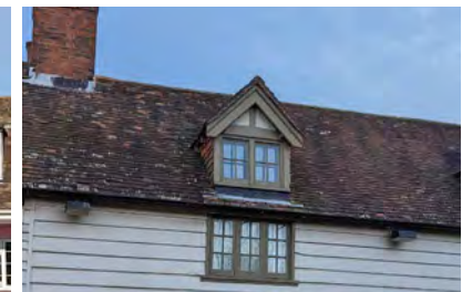
Figure 30: Kentish peg tiles and pitched roof dormers .
