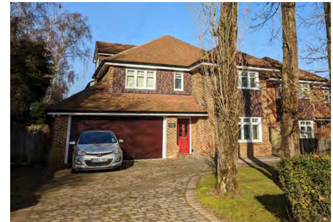
Figure 53: Local example of garage parking and permeable paving in driveway.
