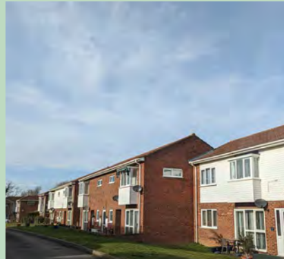
Figure 12: Houses are organised in blocks centred around open green spaces and car parking courts.
