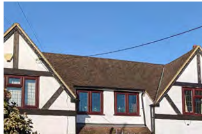
Figure 23: Cross-gabled roof with clay tiles.
