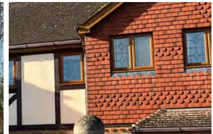
Figure 39: Hung clay tiles with variations & timber frames with white infills.
