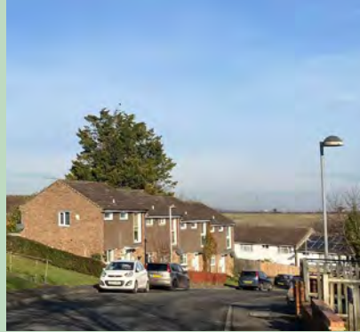
Figure 20: The hilly topography in the Wellfield Estate and the layout of the buildings allow for long views towards the open fields to the north, Caxton Close.
