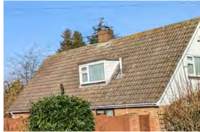
Figure 22: Gabled roof with clay pantiles, a flat dormer window and brick chimney.
