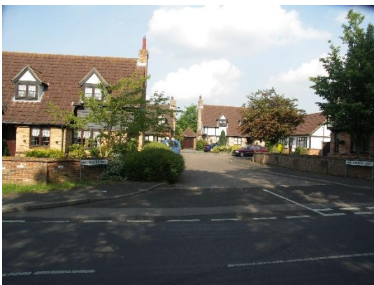
Wickhams Way (off Church Road)
