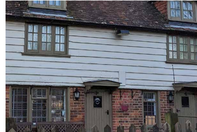
Figure 35: White weatherboarding & red brick.
