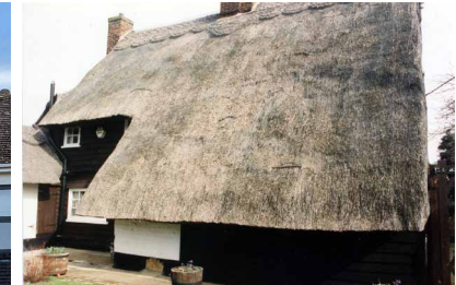
Figure 29: Hartley Cottage thatched cat slide roof.
