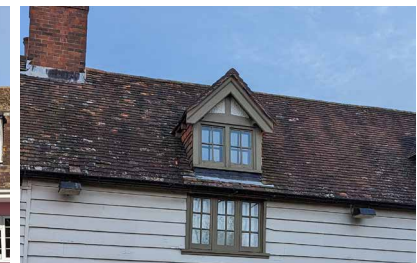
Figure 30: Kentish peg tiles and pitched roof dormers.
