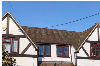
Figure 23: Cross-gabled roof with clay tiles.
