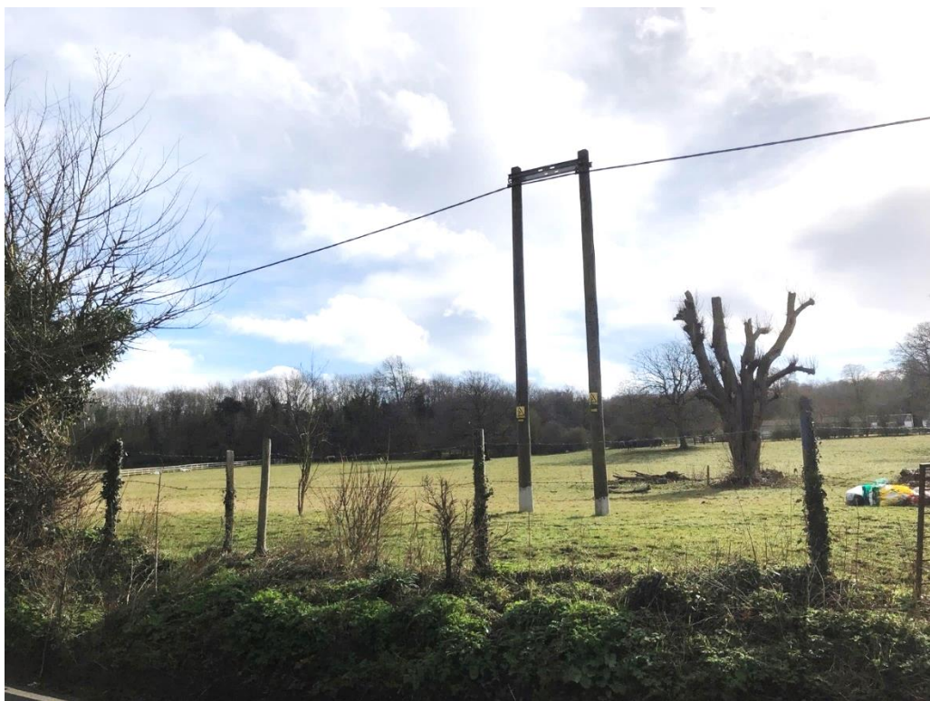
Grange Park Farm viewed from Valley Road
